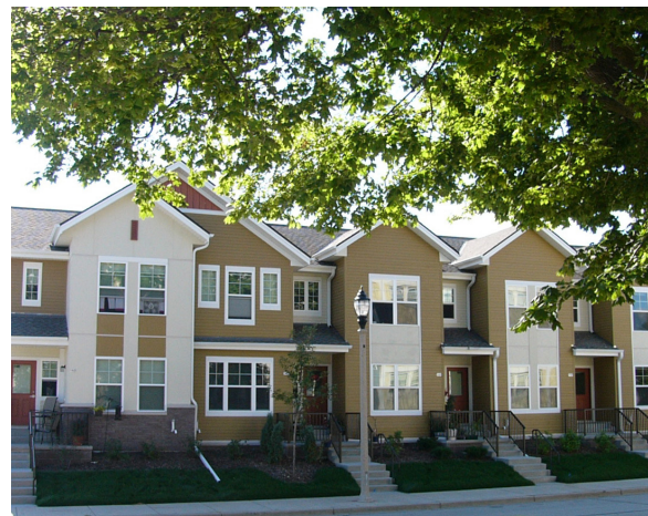
The regional housing plan recommends that local governments with sanitary sewer service ensure their comprehensive plans and zoning ordinances address the need for additional affordable housing for lower- and moderate-income households.
